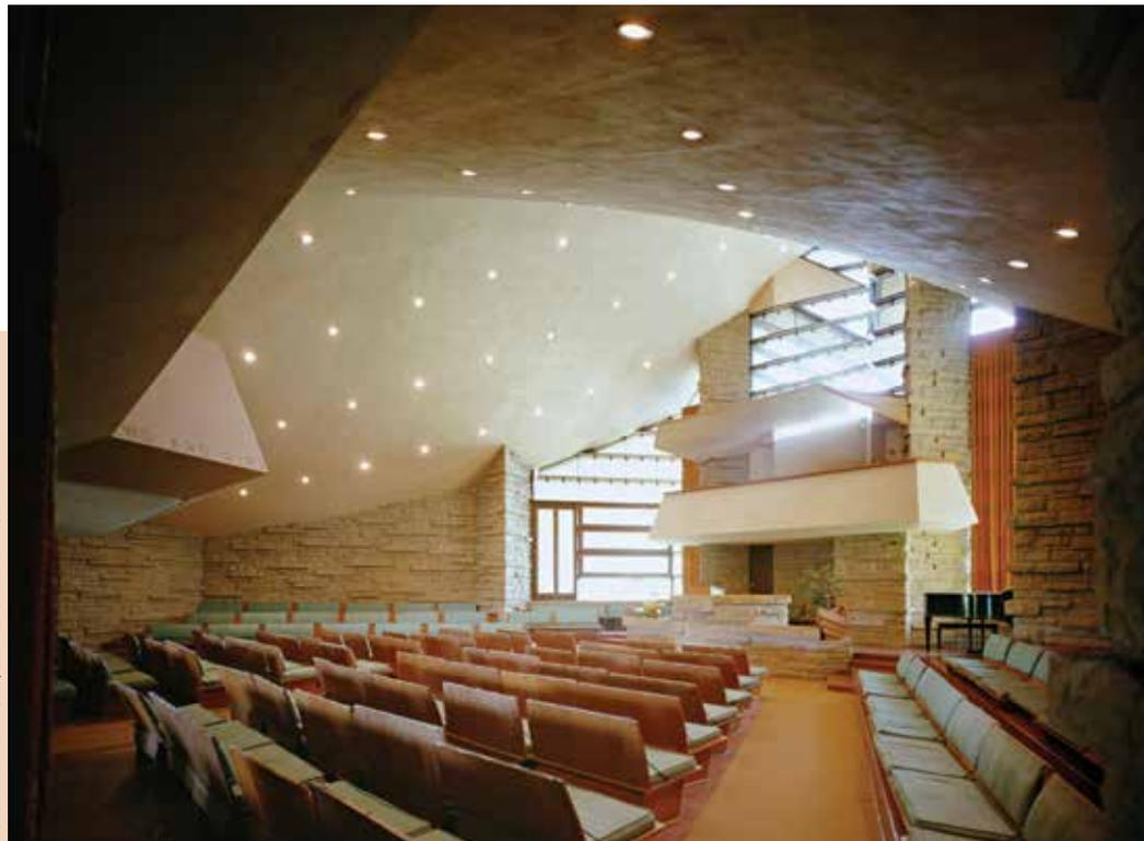
First Unitarian Society of Madison, interior view looking north toward pulpit showing plastered ceiling beneath underside of roof trusses, photographed in 1991.
