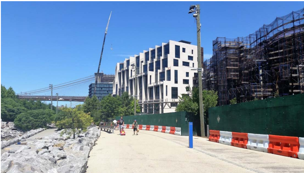
Brooklyn Bridge Park residential development underway; Personal photograph, June 2016
